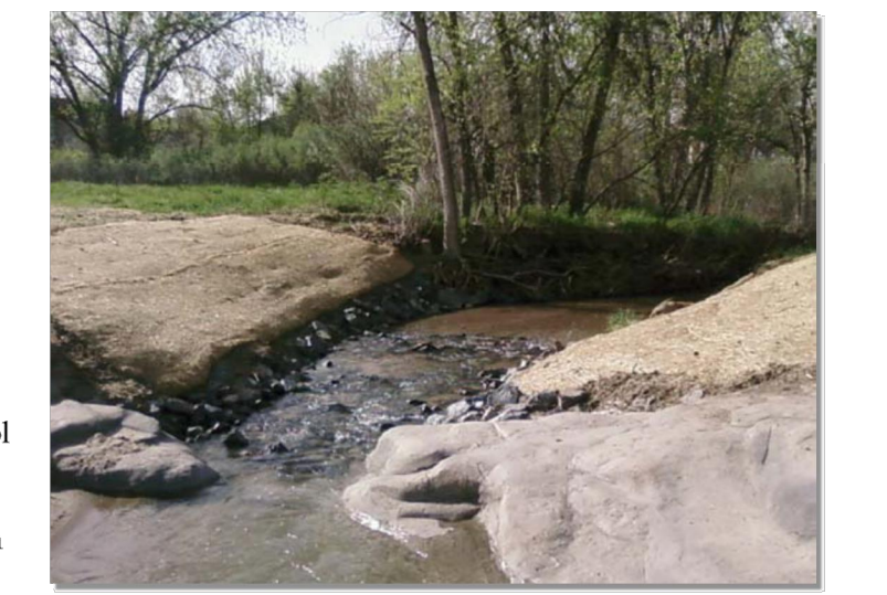
Photograph SS-1. Streambank stabilization using geotextiles following installation of a permanent in-stream grade control structure.
