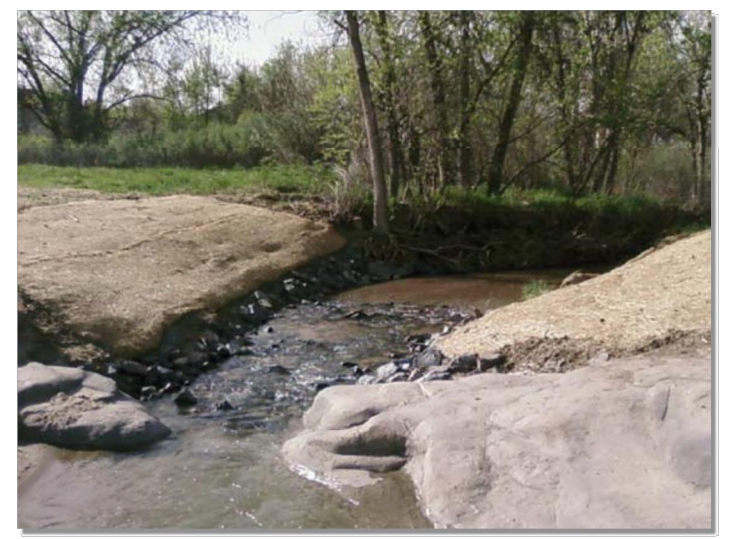
Photograph SS-1. Streambank stabilization using geotextiles following installation of a permanent in-stream grade control structure.
