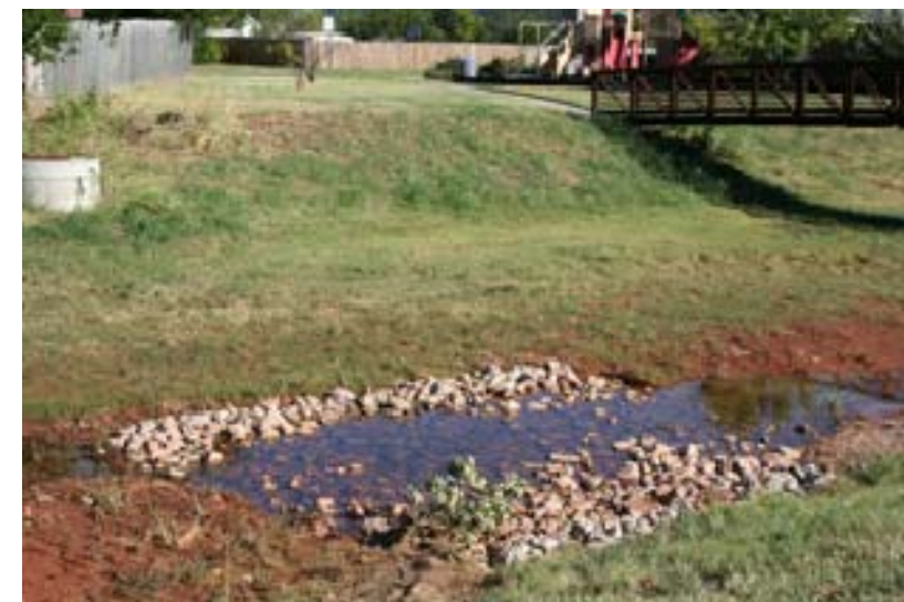
CONSTRUCTED RIFFLE DROP STRUCTURE
