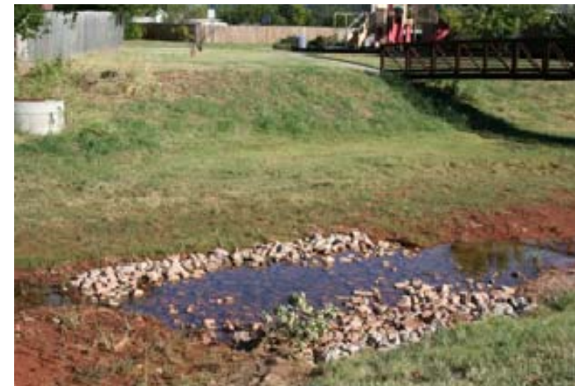
CONSTRUCTED RIFFLE DROP STRUCTURE
