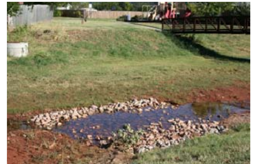
CONSTRUCTED RIFFLE DROP STRUCTURE
