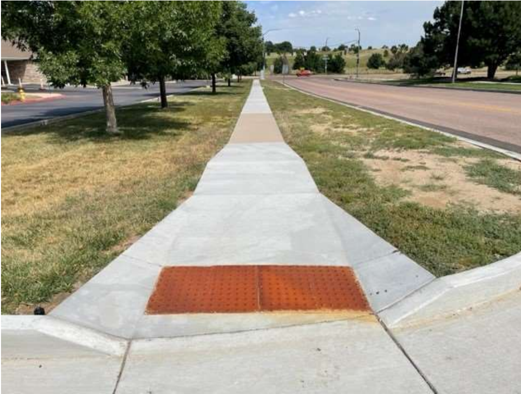
As-Built Sidewalk along Crawford Ave. facing east from site access drive
