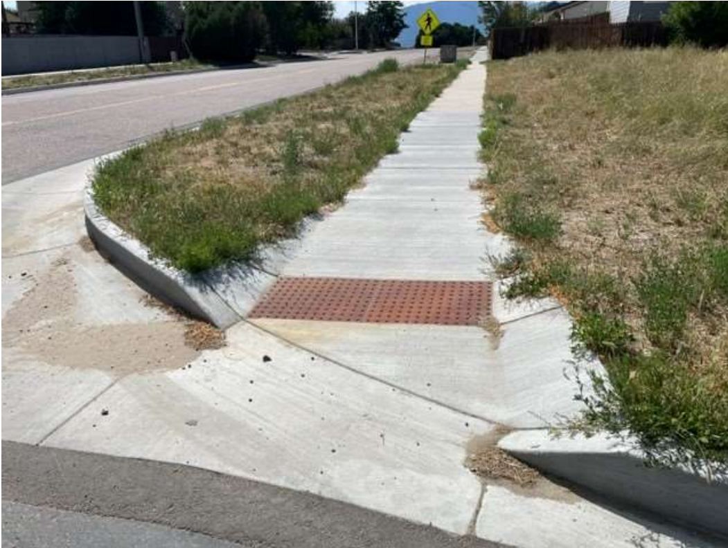
As-Built Sidewalk along Crawford Ave. facing west from site access drive
