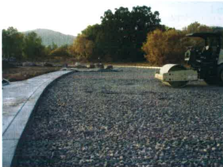
Photograph PPS-1. The reservoir layer of a permeable pavement provides storage volume for the WQCV. Photo courtesy of Muller Engineering and Jefferson County Open Space.
