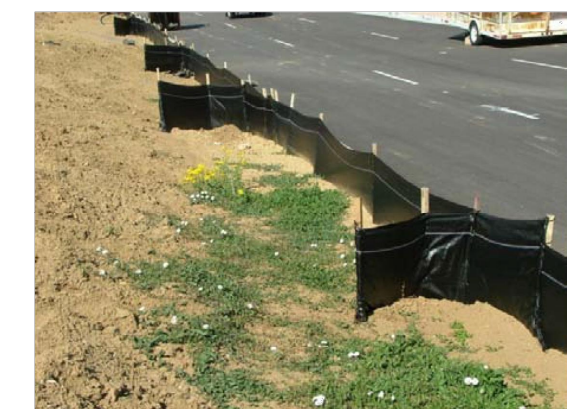
Photograph SF-2. When silt fence is not installed along the contour, a "J-hook" installation may be appropriate to ensure that the BMP does not create concentrated flow parallel to the silt fence. Photo courtesy of Tom Gore.
