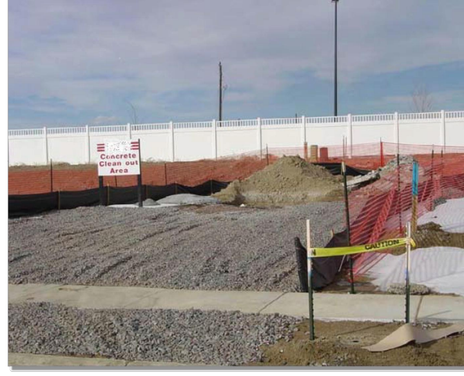
Photograph CWA-1. Example of concrete washout area. Note gravel tracking pad for access and sign.
