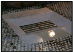
CDOT Type D Inlet Parallel (Flat & Depressed)
