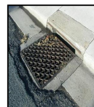
Rebarline Riveted Grate
