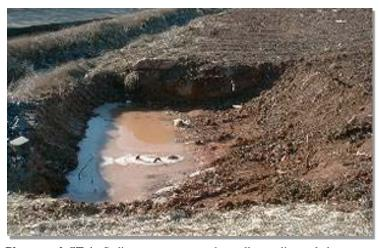
**Photograph ST-1.** Sediment traps are used to collect sediment-laden runoff from disturbed area. Photo courtesy of EPA Menu of BMPs.
