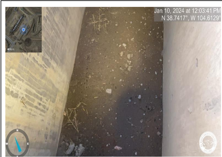
Photo 1: Clean inlets of sediment and debris.
