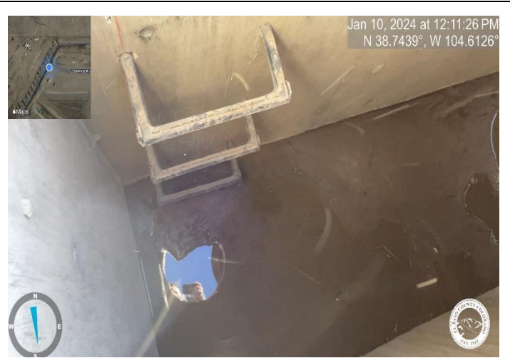
Photo 2: Clean inlets of sediment and debris.
