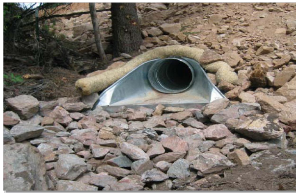
Photograph TOP-1. Riprap outlet protection.
