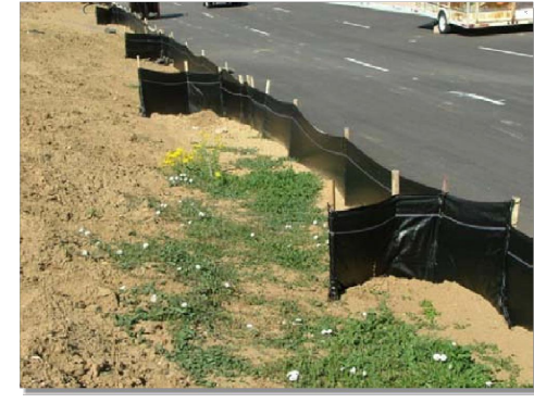
Photograph SF-2. When silt fence is not installed along the contour, a "J-hook" installation may be appropriate to ensure that the BMP does not create concentrated flow parallel to the silt fence. Photo courtesy of Tom Gave.
