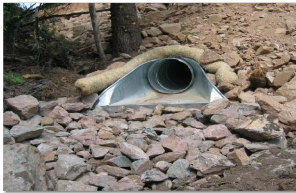
Photograph TOP-1. Riprap outlet protection.
