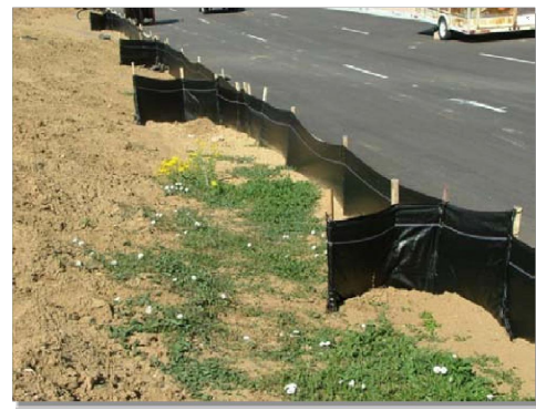
Photograph SF-2. When silt fence is not installed along the contour, a "J-hook" installation may be appropriate to ensure that the BMP does not create concentrated flow parallel to the silt fence. Photo courtesy of Tom Gave.
