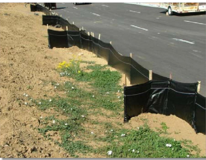
Photograph SF-2: When silt fence is not installed along the contour, a "J-hook" installation may be appropriate to ensure that the BMP does not create concentrated flow parallel to the silt fence. Photo courtesy of Tom Goss.
