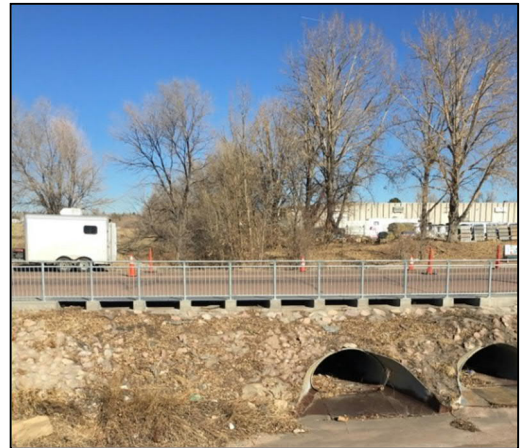
Figure 1: Existing Drainage Structures at Galley Road (Viewed from South)
