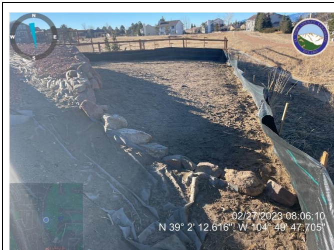
Photo 1: Finish landscaping/final stabilizing at bare areas at rear of lot. It is recommended to leave straw wattles in place until adequate vegetation is present.
