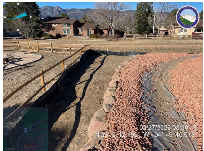
Photo 2: Finish landscaping/final stabilizing at bare areas at rear of lot. It is recommended to leave straw wattles in place until adequate vegetation is present.
