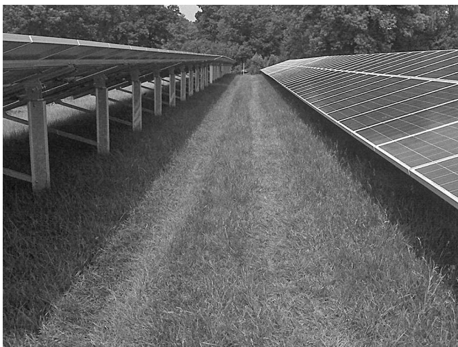
Fig. 1. Maintenance or “spacer” section between two rows of solar panels (photo by John E. Showler, reprinted with permission)
