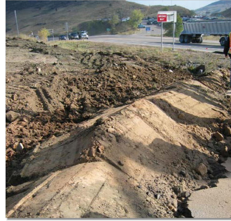
Photograph ED/DS-1. Example of an earth dike used to divert flows at a construction site. Photo courtesy of CDOT.
