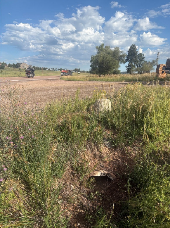
Image 2: Existing 24" CMP culvert at Highway 83 driveway (Ex DP8, Pr DPO)
