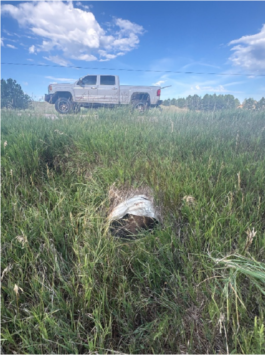
Image 10: Highway 83 existing 84" CMP culvert (Ex DP1, Pr DPB)
