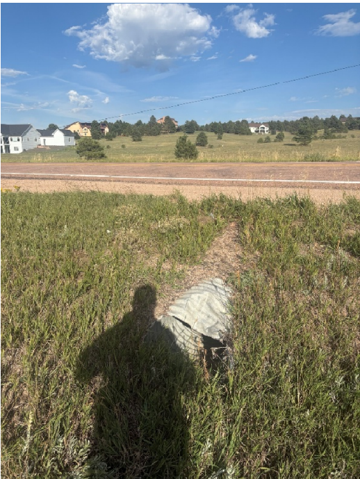
Image 2: Existing 24" CMP culvert at Highway 83 driveway (Ex DP8, Pr DPO)
