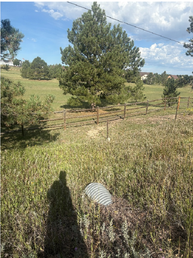
Image 12: Outfall Location - Highway 83 existing 24" CMP culvert (Ex DP3, Pr DPG)
