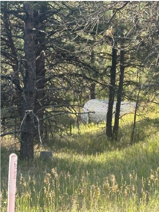
Image 10: Highway 83 existing 84" CMP culvert (Ex DP1, Pr DPB)
