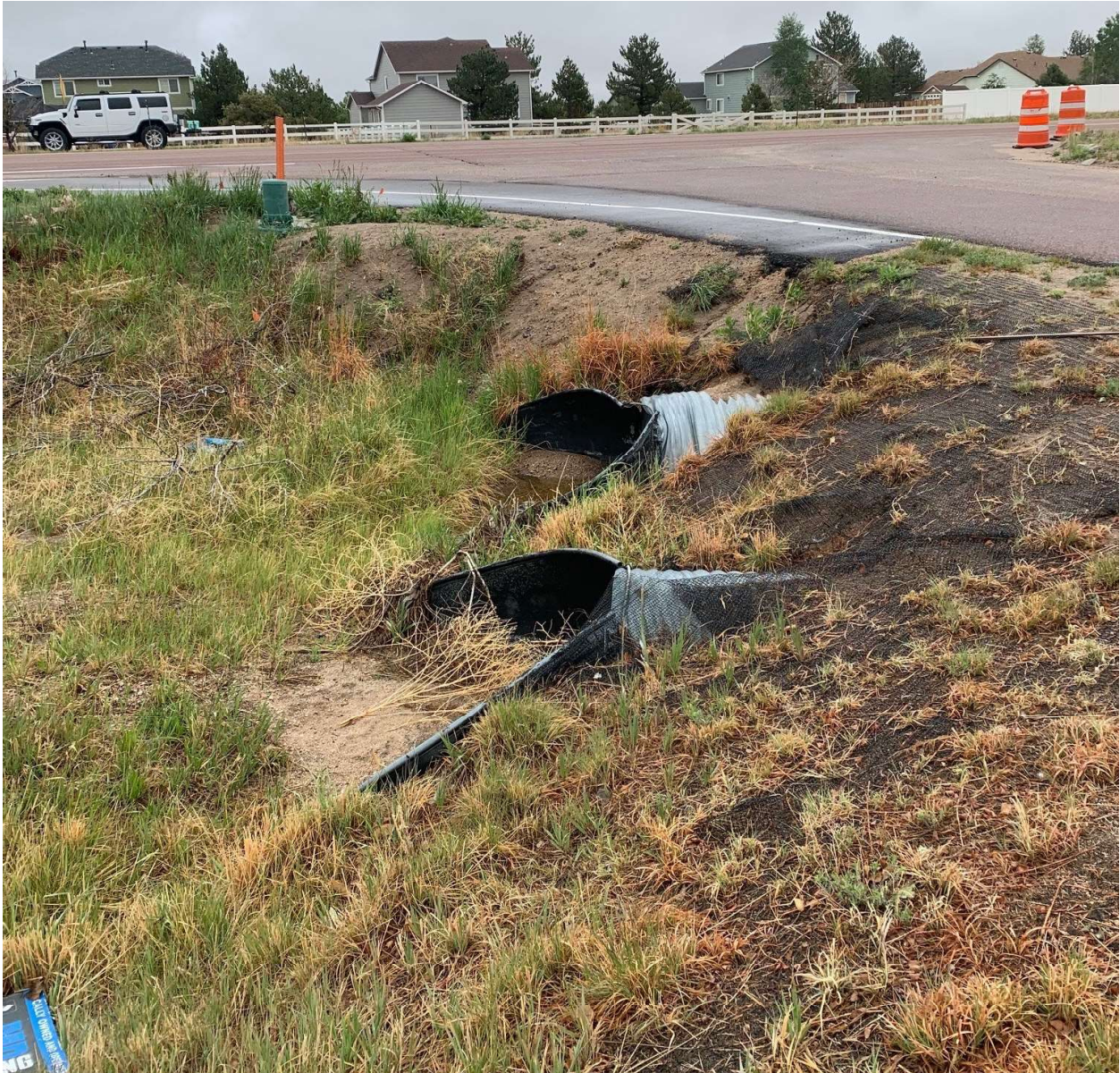
Existing 2-36" CMP under Owl Place (Upstream Inlets)
