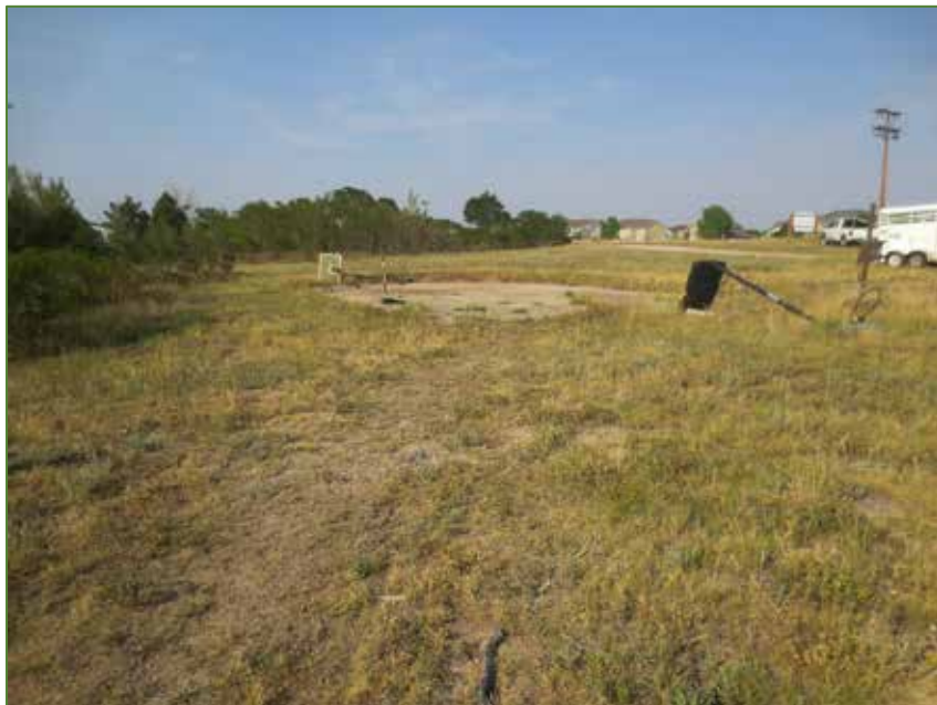
The concrete slab with broken basketball hoops/poles.
