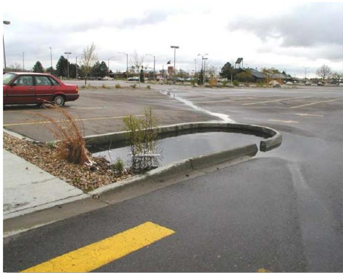
**Photograph B-4.** Runoff passed the upgradient rain garden, shown in Photo B-3, and flooded this downstream rain garden.
