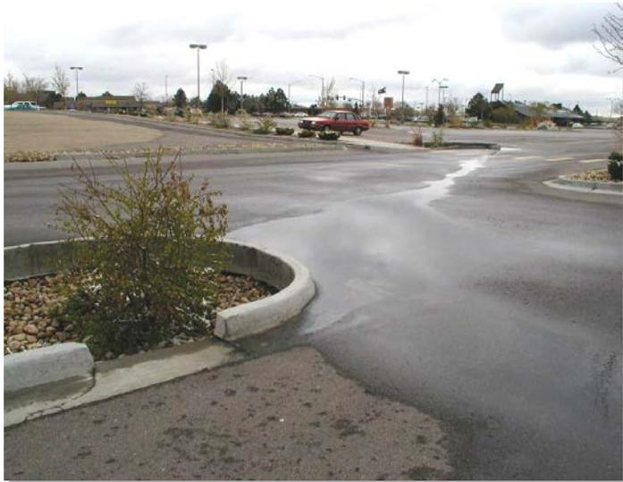
**Photograph B-3.** Inadequate construction staking may have contributed to flows bypassing this rain garden.
