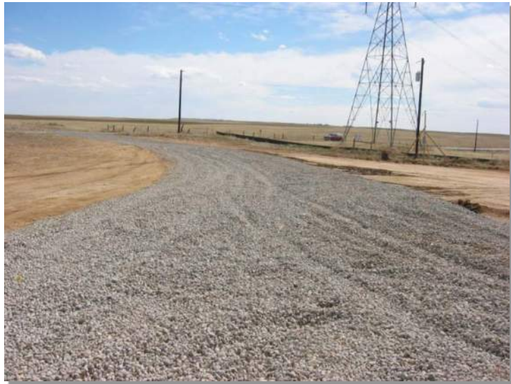
Photograph SCR-1. Stabilized construction roadway.
