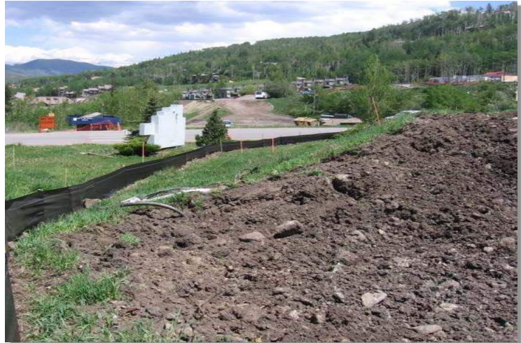
Photograph SP-1. A topsoil stockpile that has been partially revegetated and is protected by silt fence perimeter control.
