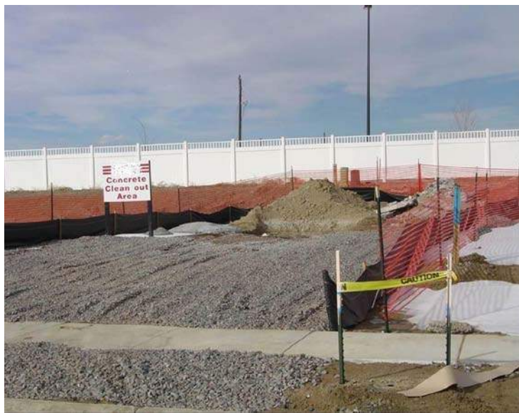
Photograph CWA-1. Example of concrete washout area. Note gravel tracking pad for access and sign.
