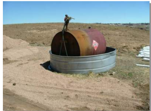
Photographs GH-1 and GH-2. Proper materials storage and secondary containment for fuel tanks are important good housekeeping practices. Photos courtesy of CDOT and City of Aurora.
