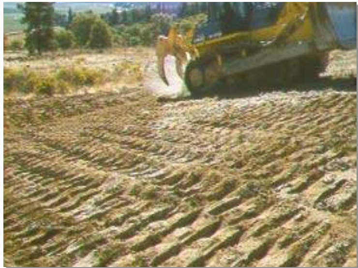
Photograph SR-1. Surface roughening via imprinting for temporary stabilization.
