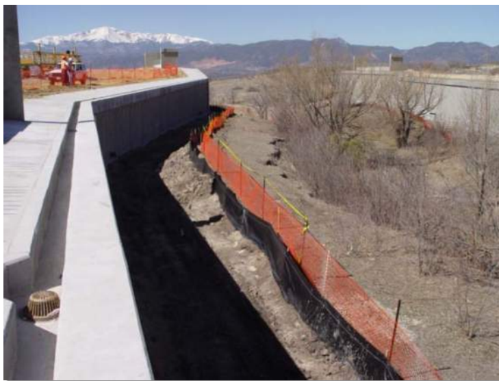
Photograph PV-1. Protection of existing vegetation and a sensitive area. Photo courtesy of CDOT.
