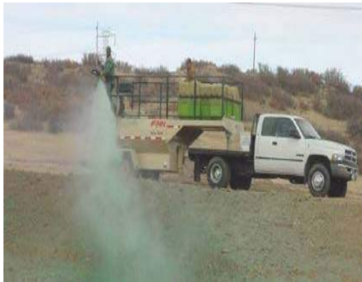
Photograph SB-1. Tackifier being applied to provide temporary soil stabilization. Photo courtesy of Douglas County.
