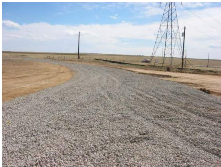
Photograph SCR-1. Stabilized construction roadway.
