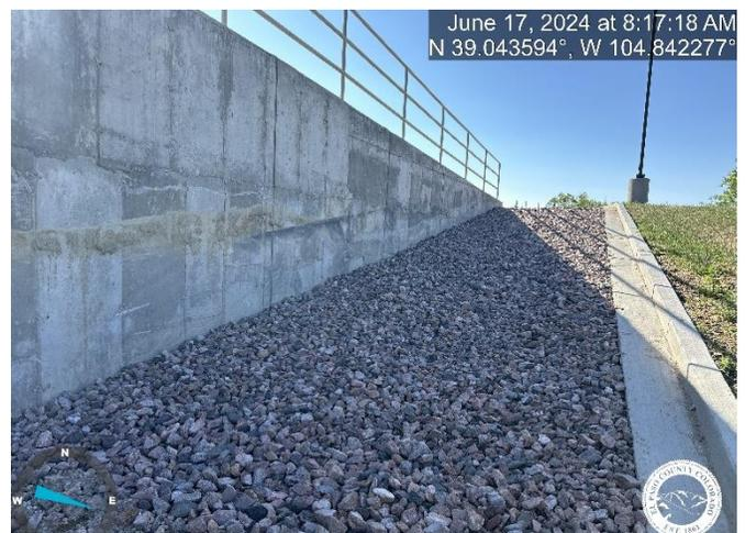
**Photo 4:** Plans call for Class 5 or 6 road base. 2-4" stone was installed. Show on as-builts.
