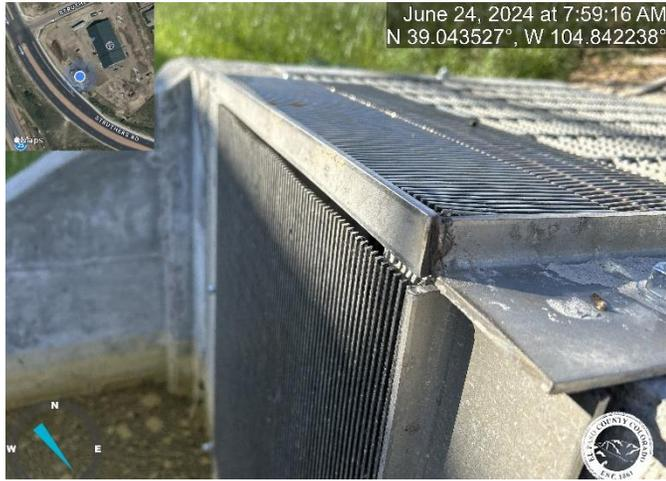
**Photo 5:** 12" Concrete opening width is covered with Johnson Vee Wire with 1/2" gap. Show on as-builts.
