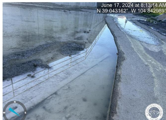
**Photo 3:** Trickle Channel: Appears to be about 1" in depth. Plans call for 6". Fill in pond bottom to match top of trickle channel.
