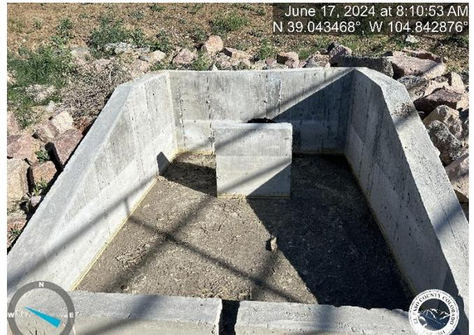
**Photo 2:** Dissipator Baffle: Is 2'Lx2'H. Plans call for 3'Lx2'H.
