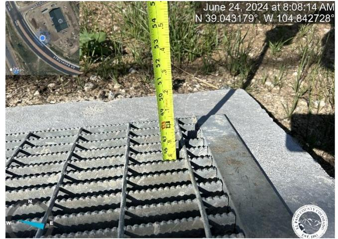
**Photo 6:** Outfall structure is 3'9" tall, as opposed to 6' on the plans. Install per approved plans or confirm with your project engineer that this change from the plans is acceptable and then reflect the change on the as-builts.
