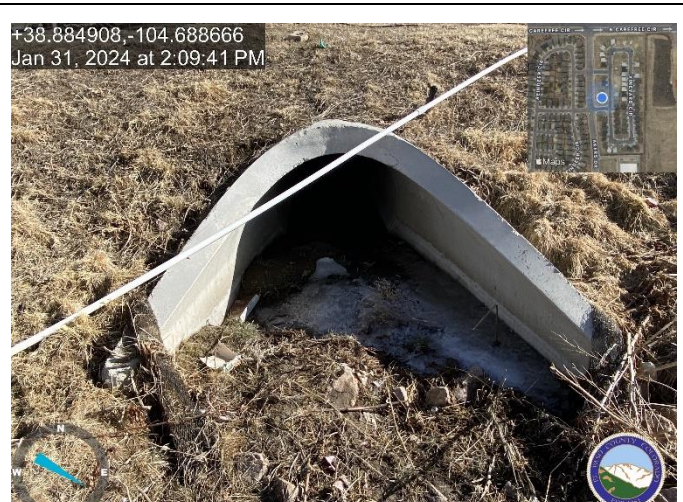
Photo 4: Remove sediment from flared end section. (North Pond)
