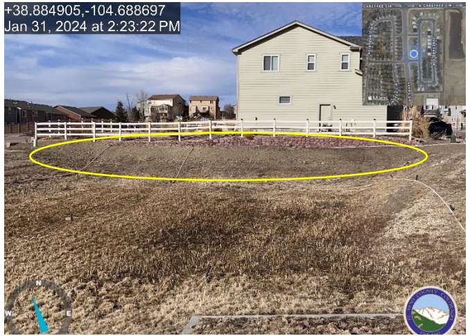
Photo 6: Stabilize northern pond embankment at north pond.
