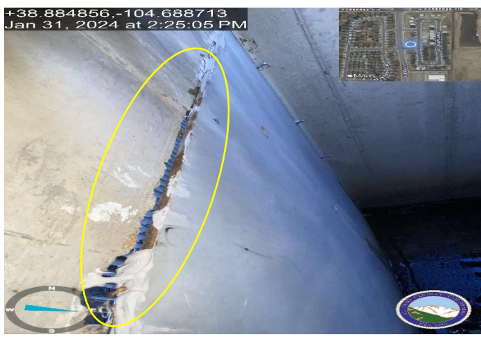
Photo 7: Re caulk orifice plate at outlet structure.
