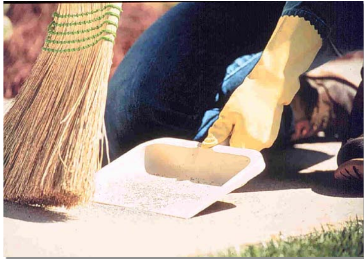
Photograph GH-1. Use dry clean-up methods to remove spilled materials. Photo courtesy of Colorado Nonpoint Source Program.
