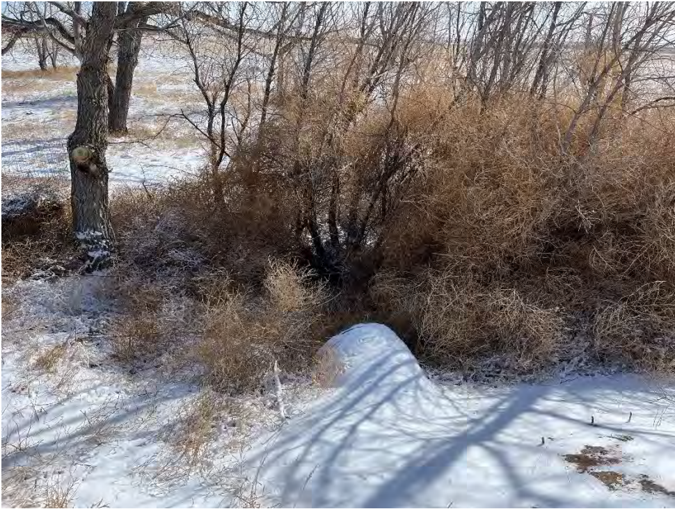
48" CMP at North Log Road Crossing (downstream of project, looking east)
