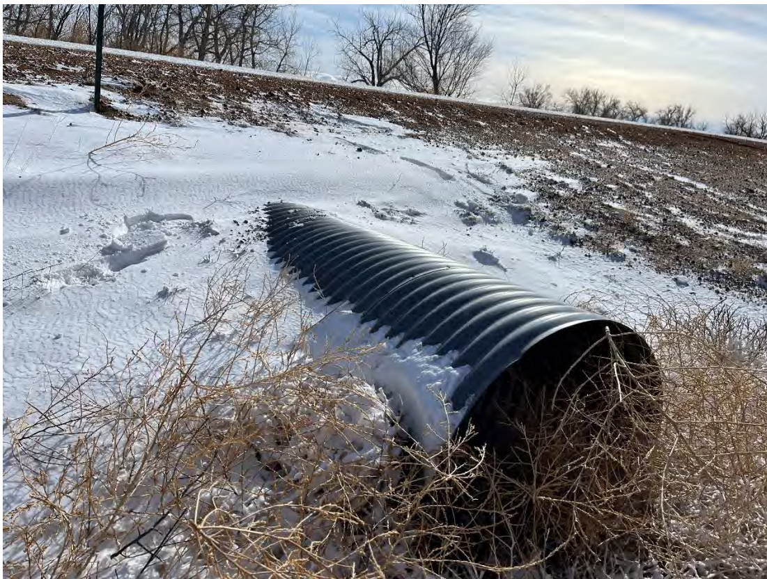
48" CMP at North Log Road crossing (downstream of project, looking west)
