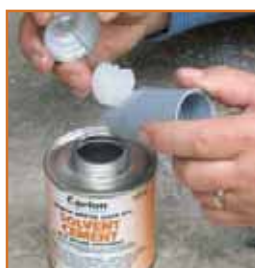
Apply a uniform coat of cement.
