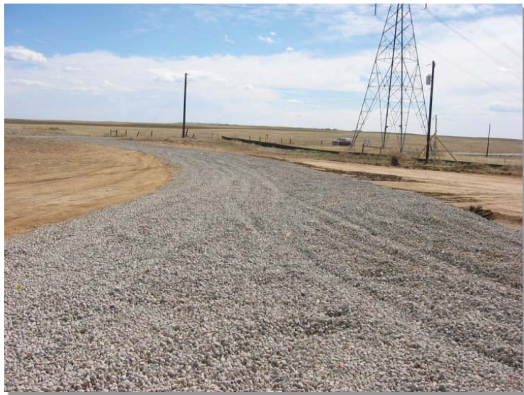
Photograph SCR-1. Stabilized construction roadway.
