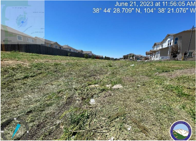
Photo 6: Clear and remove vegetative debris from swale upstream of pond.
