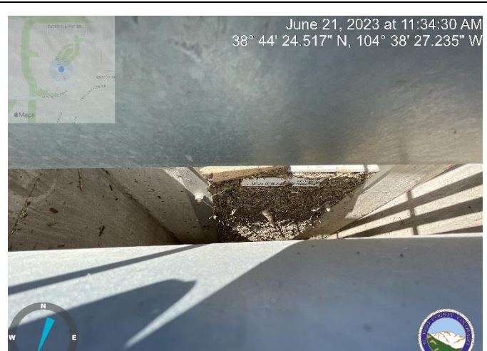
Photo 4: Outlet structure microscreen. Remove debris.
