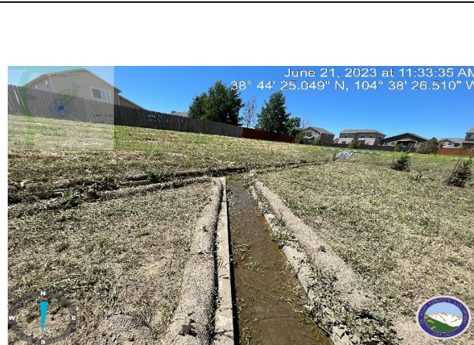
Photo 3: Clean out low flow channel of sediment and debris throughout structure.
