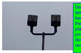
Several existing lamp fixtures has been tilted above the horizontal plane. Light is not projected downward as required
