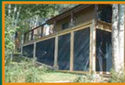
Figure 16: Enclosing decks with metal screens can prevent embers from igniting a house. Photo: Marilyn Brown, La Plata County
