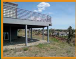
Figure 14: This homeowner worked hard to create a defensible space around the home. Notice that all fuel has been removed within the first 5 feet of the home, which survived the Waldo Canyon Fire in the summer of 2012. Photo: Christina Randall, Colorado Springs Fire Department
