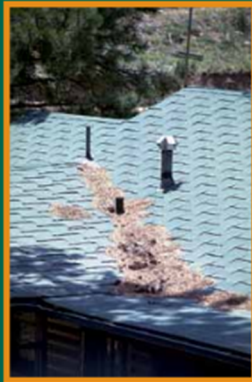
Figure 15: Clearing pine needles and other debris from the roof and gutters is an easy task that should be done at least once a year. Photo: CSFS
