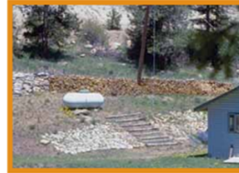
Figure 19: Keep firewood, propane tanks and natural gas meters at least 30 feet away from structures. Photo: CSFS
