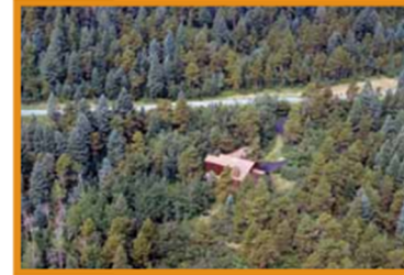
Figure 28: This house has a high risk of burning during an approaching wildfire. Modifying the fuels around a home is critical to reduce the risk of losing structures during a wildfire. Photo: CSFS
