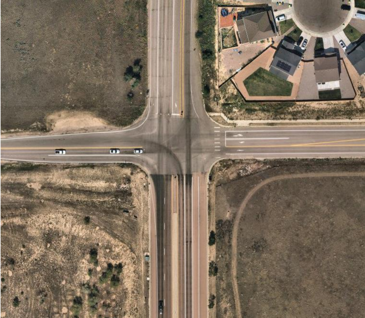
Bradley Road and Grinnell Boulevard (#5)
