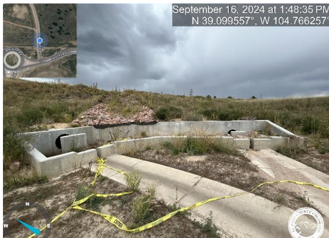
Photo 3: Clean out riprap and sediment from forebay at pond C14.
