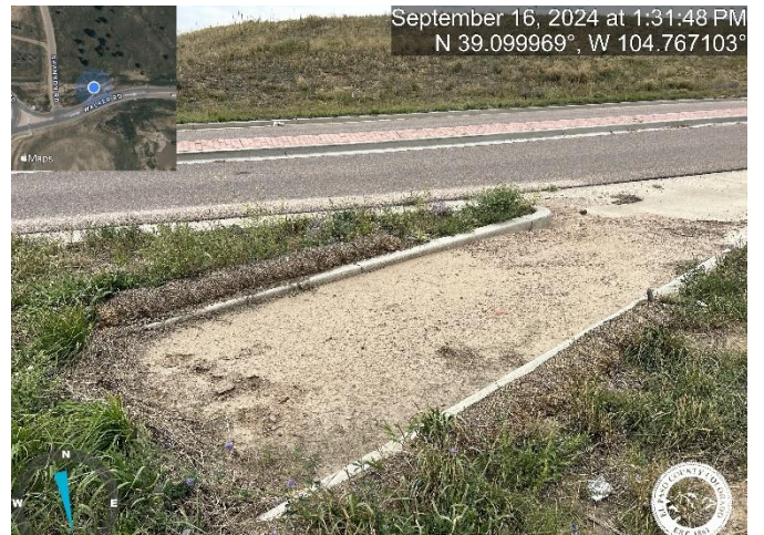
Photo 12: Clean concrete pan near Rain Garde OM2.
