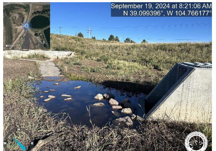
Photo 4: Regrade and re-install riprap to ensure positive drainage.
