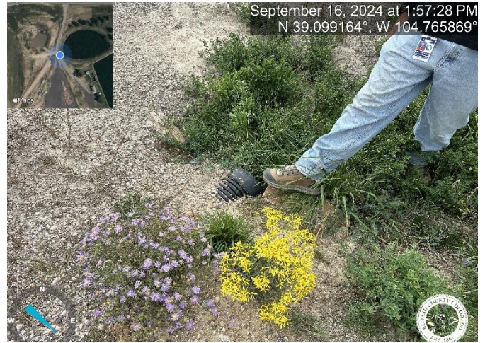
Photo 6: Clean sediment from 8" culvert pipe at maintenance road at pond C14.
