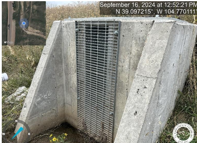
Photo 1: Install No. 93 Johnson Vee Wire stainless steel well screen and tubular trash rack.
