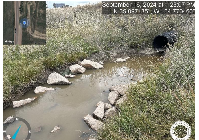
Photo 2: Re-install riprap rundown and install FES pipe to allow for positive drainage.
