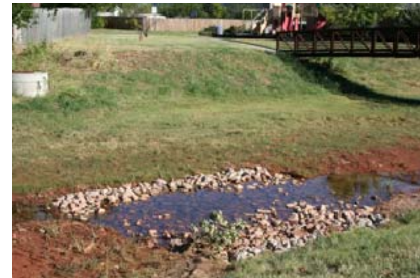
CONSTRUCTED RIFFLE DROP STRUCTURE
