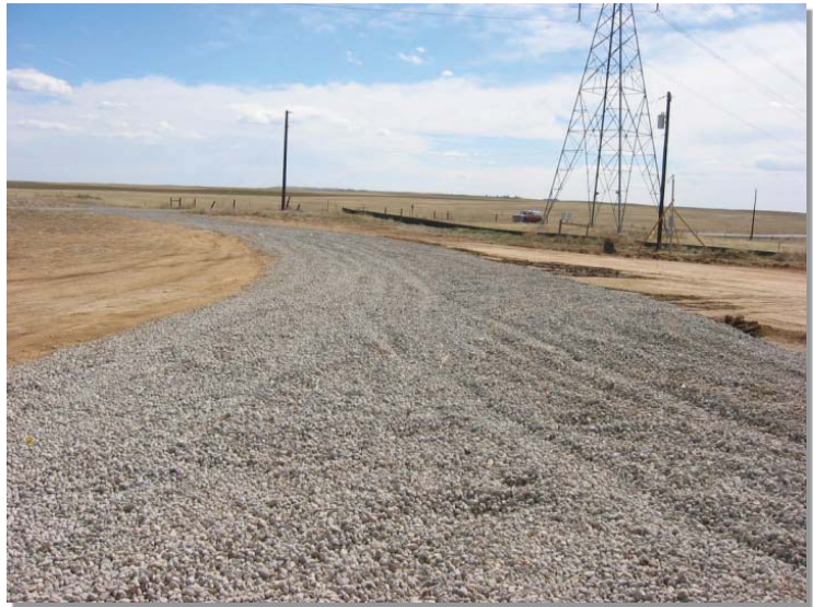
Photograph SCR-1. Stabilized construction roadway.
