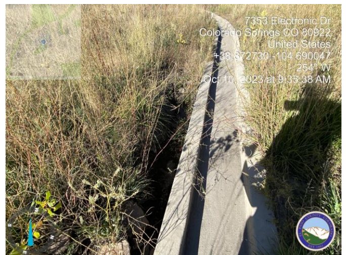
Photo 6: Address erosion near trickle channel.
