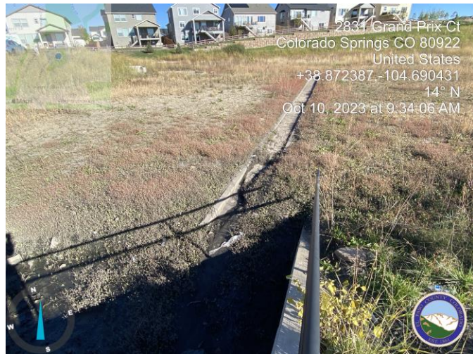
Photo 3: Trickle channel requires maintenance.
