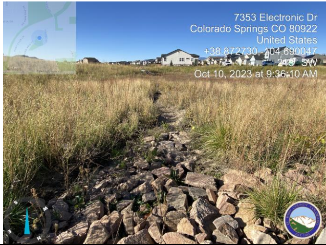
Photo 7: Address erosion near Eastern forebay and mow pond bottom
