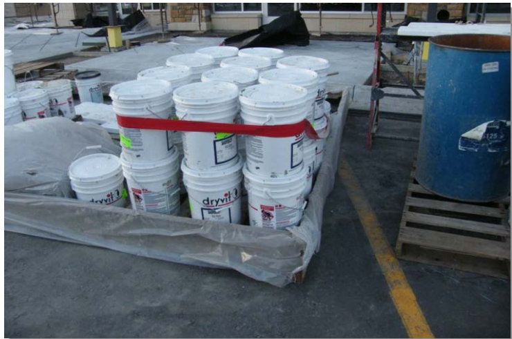
Photograph SPCC-1. Use of secondary containment around supplies stored outside helps to reduce the likelihood of spill and leaks reaching the storm sewer system in runoff. Photo courtesy of Tom Gore.
