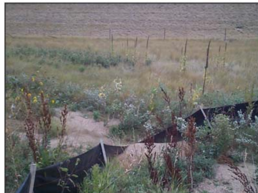
This photo illustrates what will happen to a silt fence if it is installed in an area of concentrated flow.
