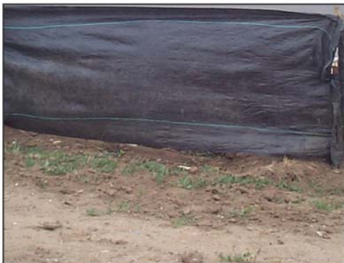
This photo reveals a silt fence that has become unentrenched because it was not securely installed.
