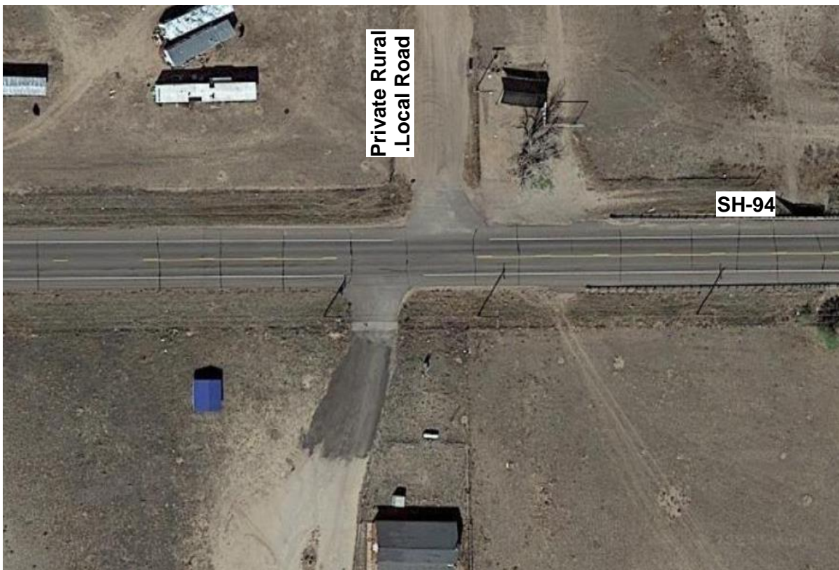
SH-94 and Private Rural Local Road
