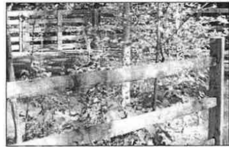
F 4' HT. WOOD POST AND RAIL FENCE NOT TO SCALE
