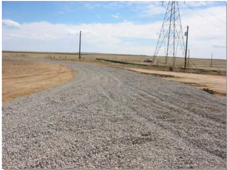
Photograph SCR-1. Stabilized construction roadway.
