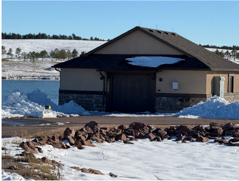
Figure 2: Pump House located at 6570 Old Stagecoach Rd.
