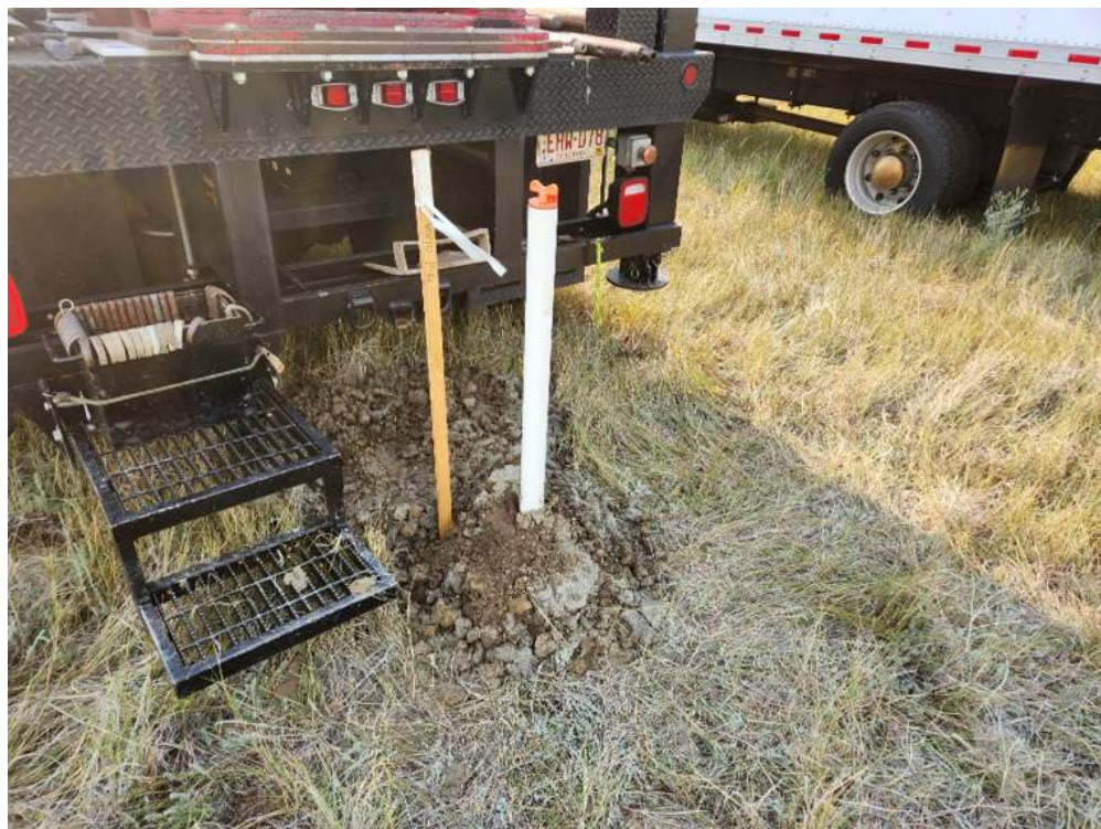
PIEZOMETER INSTALL AT BORING P-6
