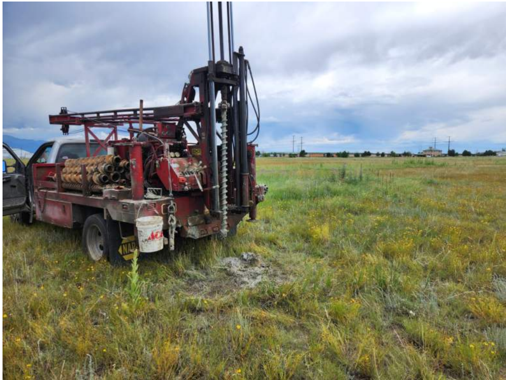
SITE CONDITIONS AT BORING B-6 - LOOKING NORTHWEST
