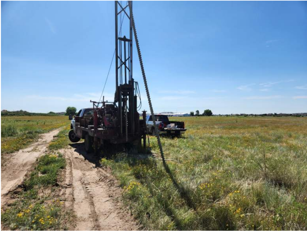
SITE CONDITIONS AT BORING B-11 - LOOKING EAST
