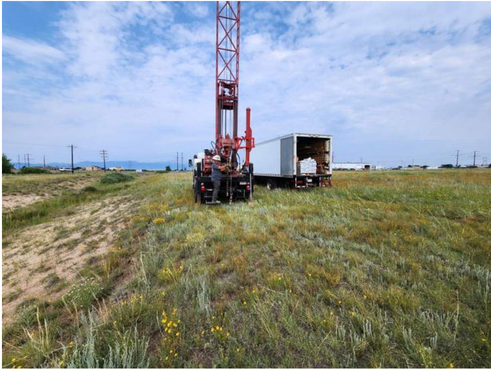
SITE CONDITIONS AT BORING P-2 - LOOKING WEST
