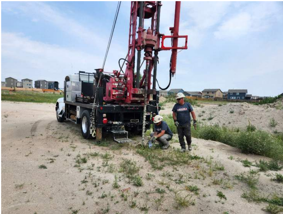
SITE CONDITIONS AT BORING B-15 - LOOKING NORTH
