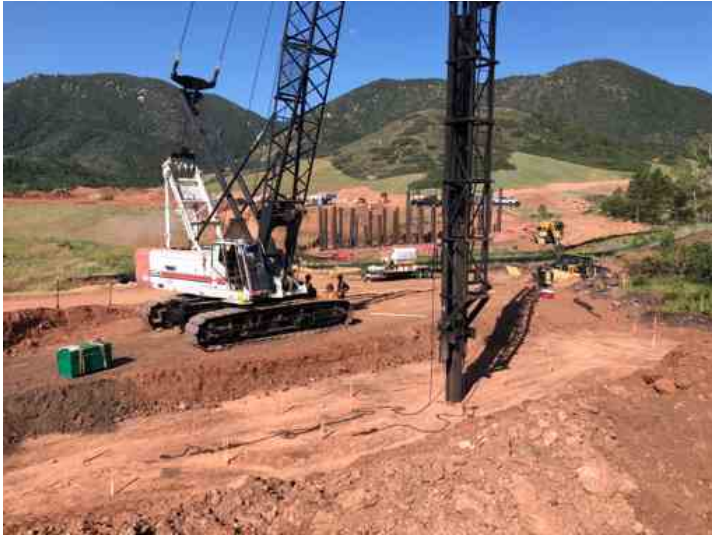
Pile driving at Abutment #3
