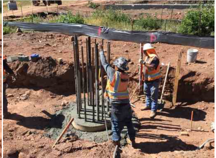
Filling of CSL tubes in WB-2
