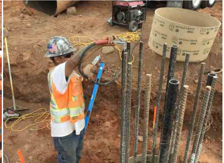
Filling CSL tubes with water
