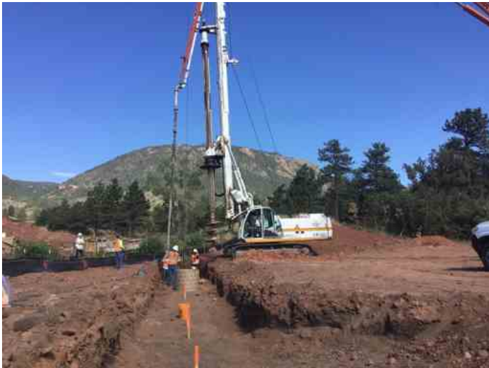
35' Long Tremmie Pipe for Concrete Placement
