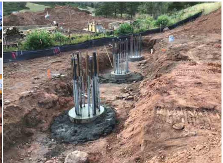
WB-3, CSL tubes filled and covered with duct tape
