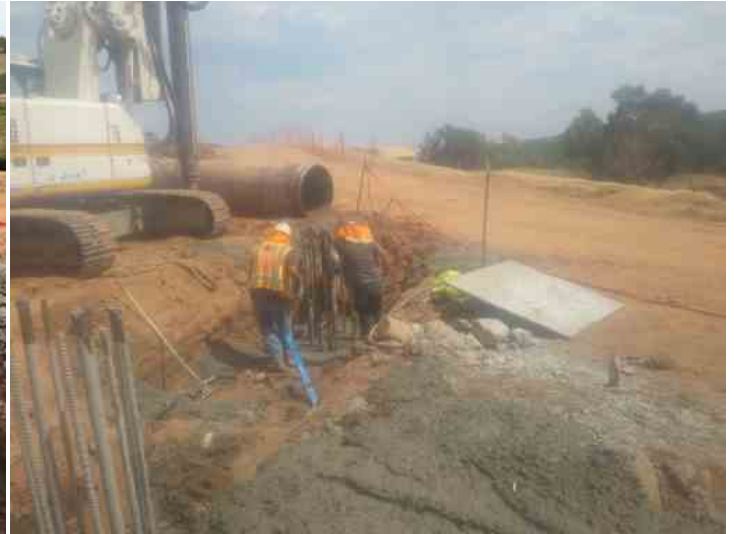
Filling of EB-3 CSL tubes prior to concrete placement
