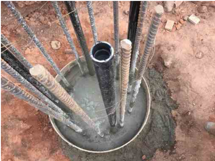
Water Level inside CSL tube
