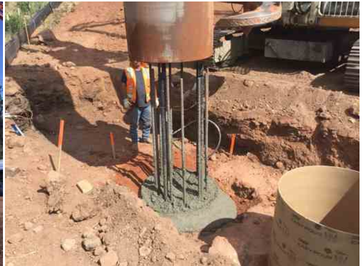
Concrete After Casing removal
