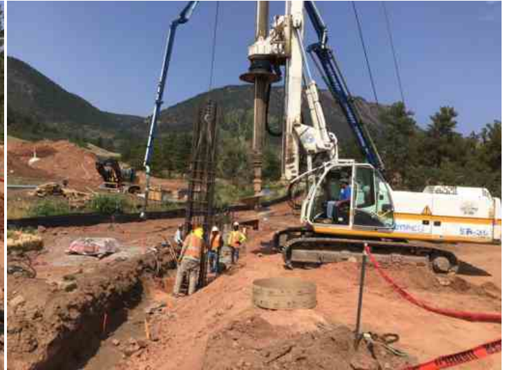
Placing rebar cage in EB-1
