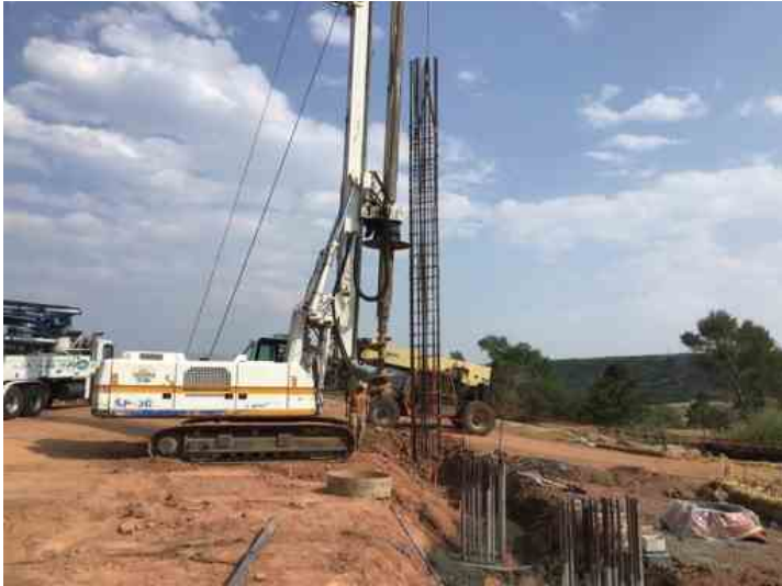
Placement of rebar cage in EB-2
