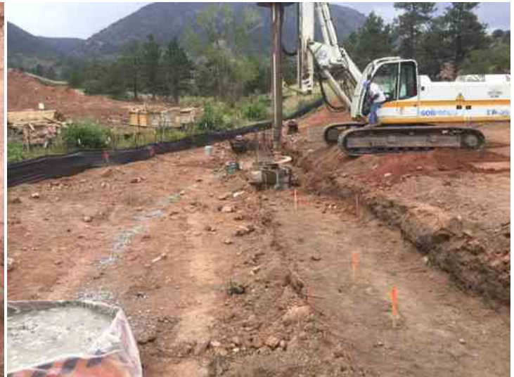
Casing Placed after Drilling Hole at Location 2
