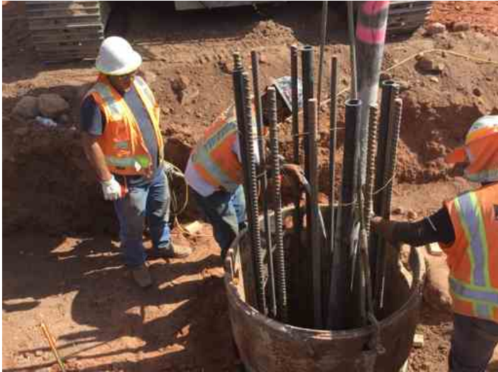
Vibrating Top 5' of Pier after concrete Placement
