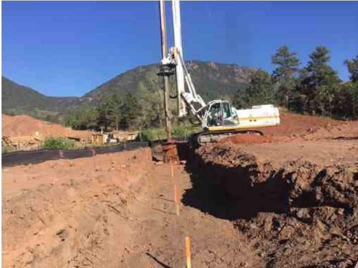
Drilling Hole for WB Pier at Location 1
