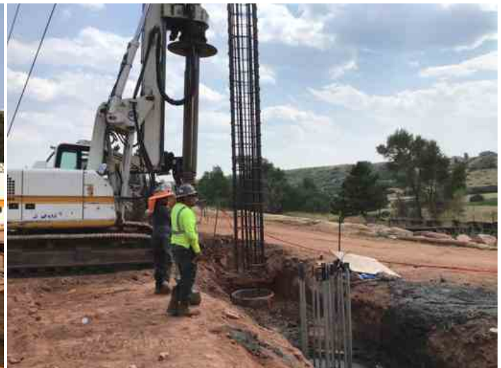
Cage placement in EB-3
