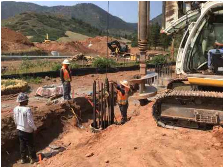
Filling of CSL tubes on EB-1 prior to concrete placement
