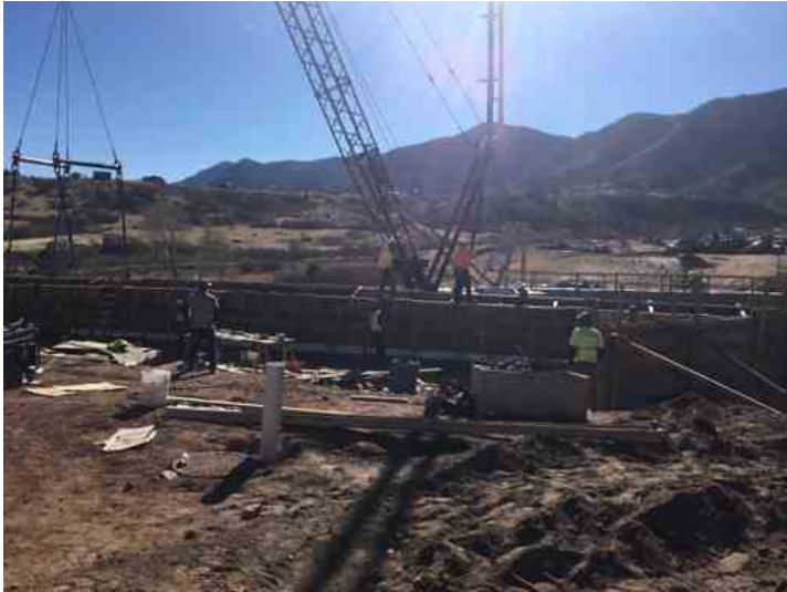
Concrete being pumped into top portion of abutment 3
