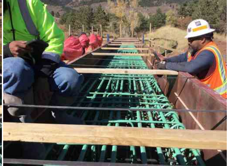
Rebar and forms on eastbound side of bridge
