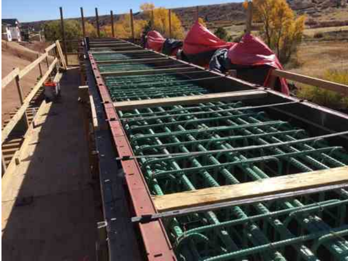
Rebar and forms on westbound side of bridge
