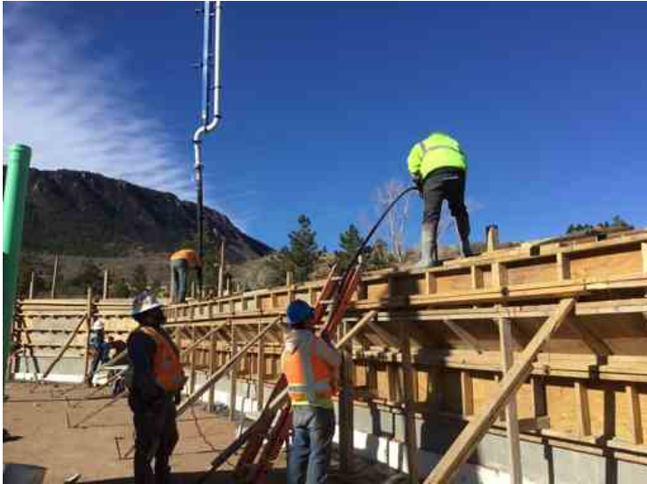
Placement of concrete for abutment
