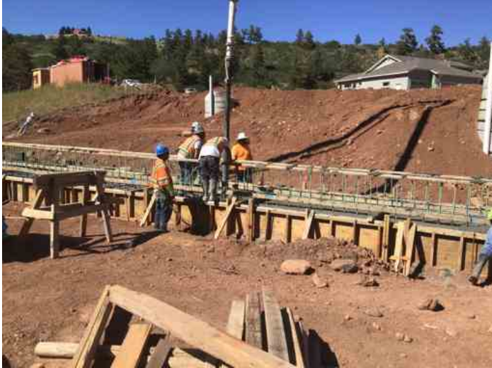
Concrete placement
