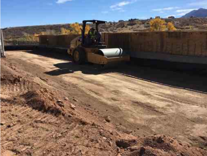
Smooth drum roller being used for compaction
